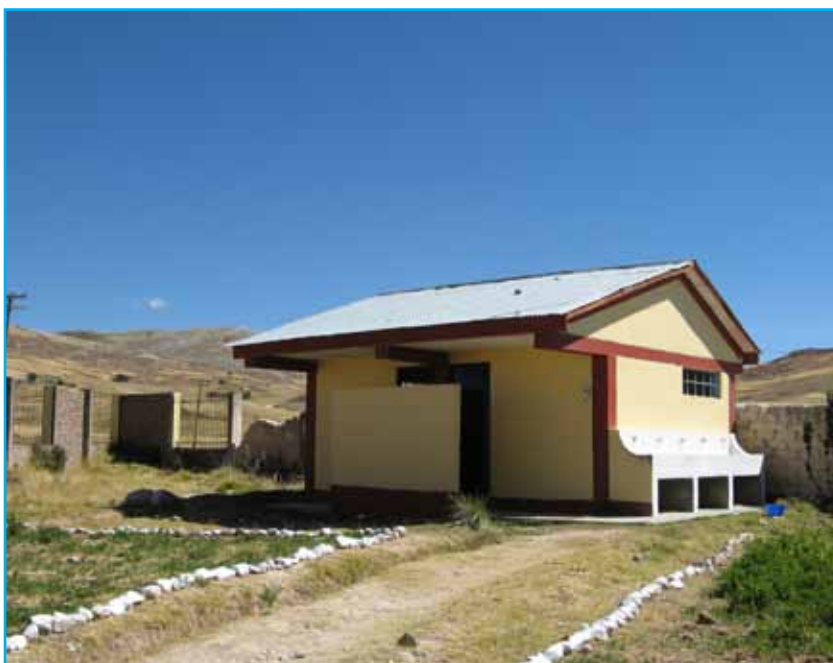
Children's toilets with a hand washing station at a school on the Alitplano.
